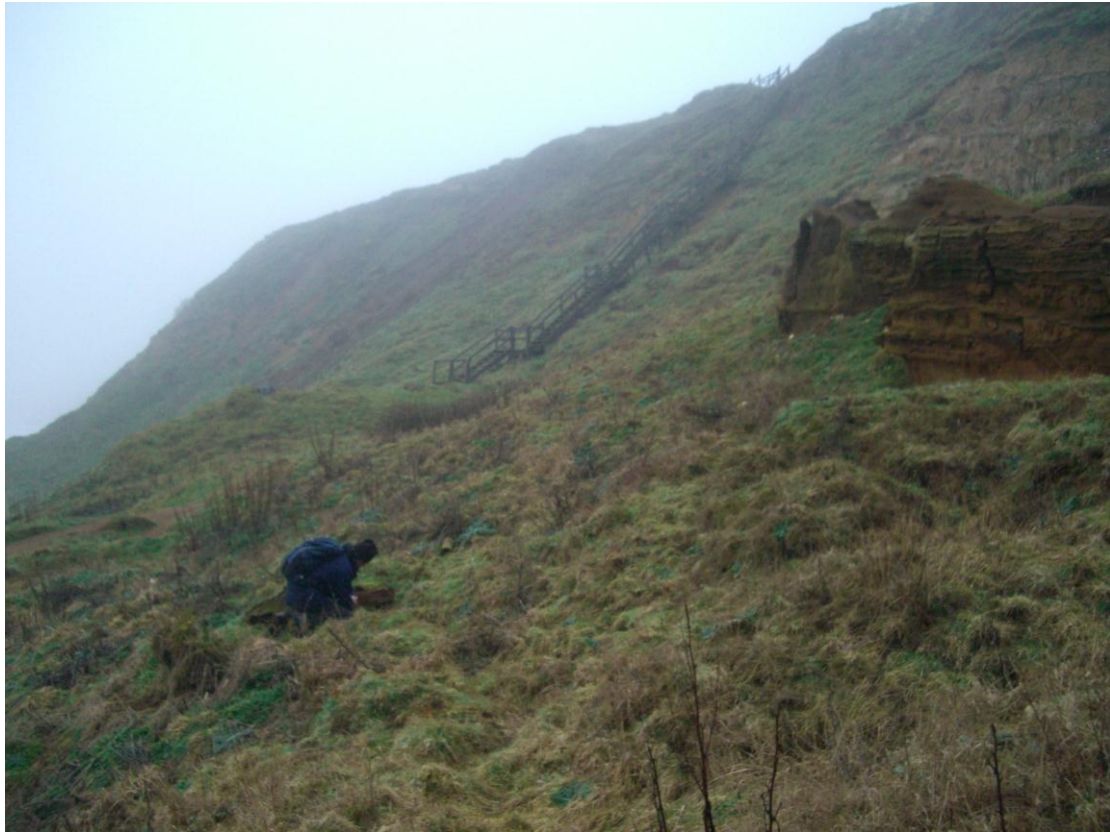
Figure 5: Vegetated landslide at Compton Bay (SZ370849)
